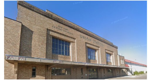
1547 Critical Systems Realty
