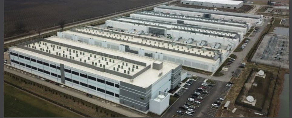
Amazon Web Services (AWS) Data Center
