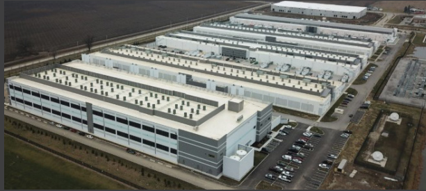
Amazon Web Services (AWS) Data Center
